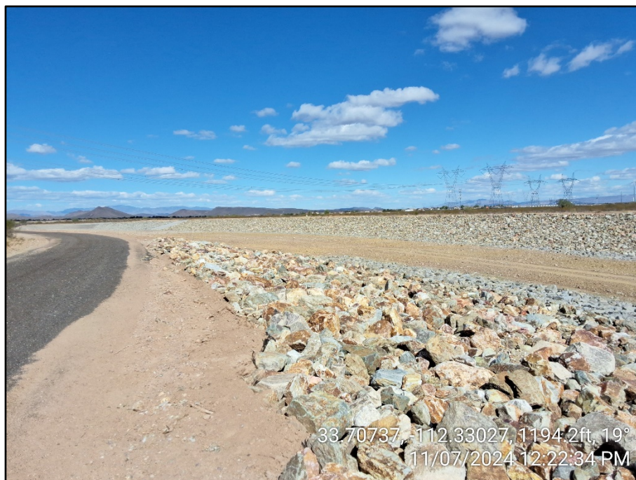
Photograph 4. Overview of McMicken Dam Outlet Channel. Photo was taken west of McMicken Dam Outlet Channel and is facing north. Note: lack of surface waters or riparian vegetation.
