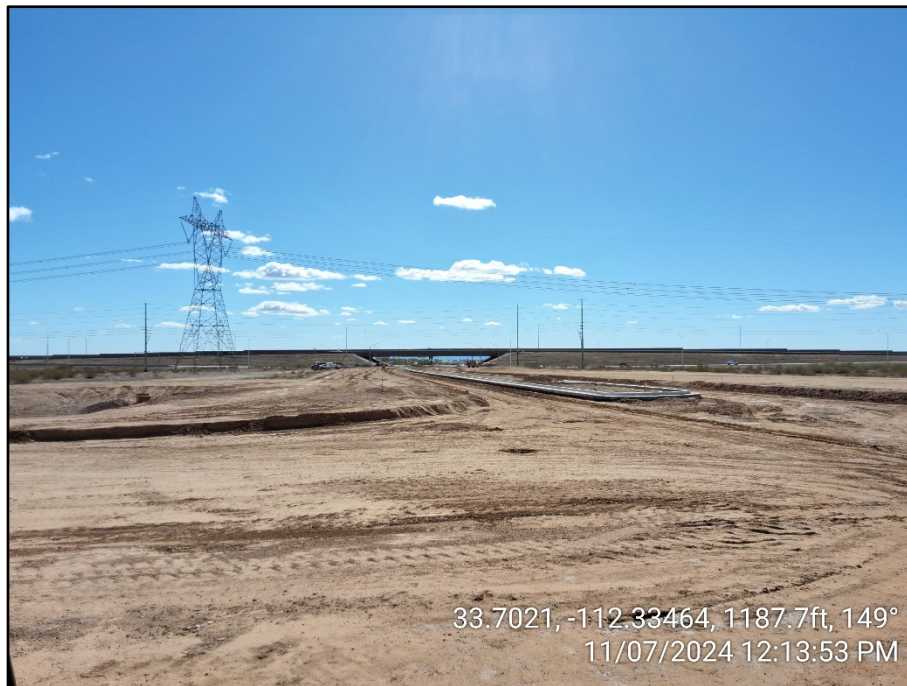
Photograph 1. Overview of the southern terminus of the project area. Photo was taken north of SR303L at the proposed road alignment, and is facing southeast.
